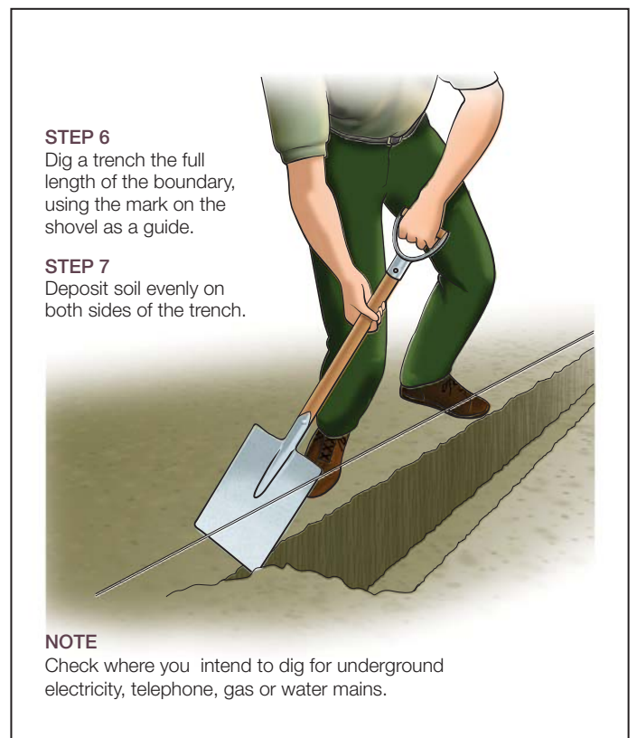
FIGURE 5 DIGGING TRENCH FOR HARDIFENCE SHEETS
